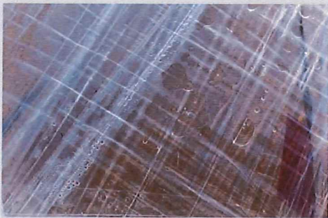
Figs 13/14 Potentially damaging condensation was clearly evident beneath the impermeable film cover
